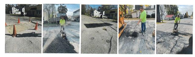
• Fed Excavating has completed the final catch basin on Lytle Road. Please let me know if you notice any deteriorating catch basins for next year's repair or replacement list.
