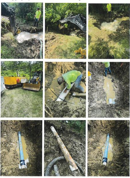
• The second waterline break was in the 900 block of Franklin Road / Old SR73. The Maintenance and Water Department worked as a team to repair the break and they will be doing property restoration and repair as soon as the ground settles.
