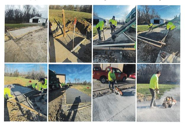
• KT Holden has completed the waterline, storm waterline, lateral lines, curbs, and handicap ramps on Franklin Road. We performed a walk-through on Wednesday, March 13<sup>th</sup> and I pointed out a few areas of concern. They are working on correcting a few items before the final paving takes place. Contingent on the weather and the asphalt plants opening, they will be repaving the street in mid-April. The grindings will be used to add surface to the Village Maintenance driveway.
